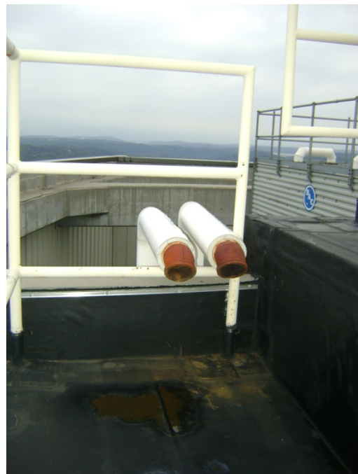
Figure 3. Exhaust Breaching at Roof – probe inserted into breaching approximately 2-feet.
