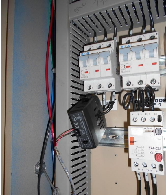
Veris H921 Analog CT on Dump Radiator
