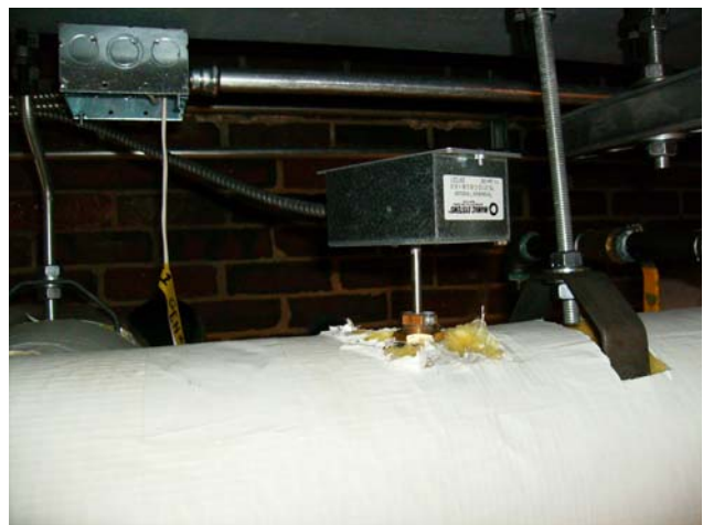
Loop Return Temperature Before Cooler (TLRBC)
