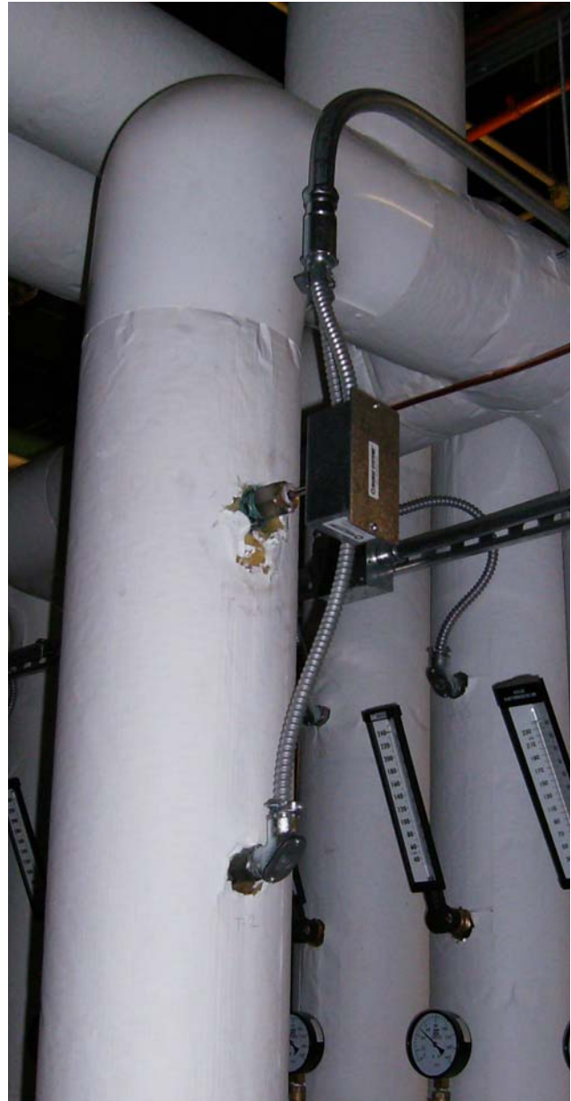
Loop Supply Temperature (TLS)
