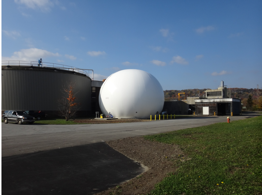
Digesters and Biogas Storage
